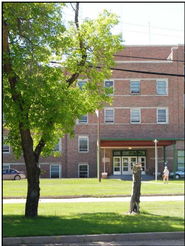
Humboldt District Hospital
